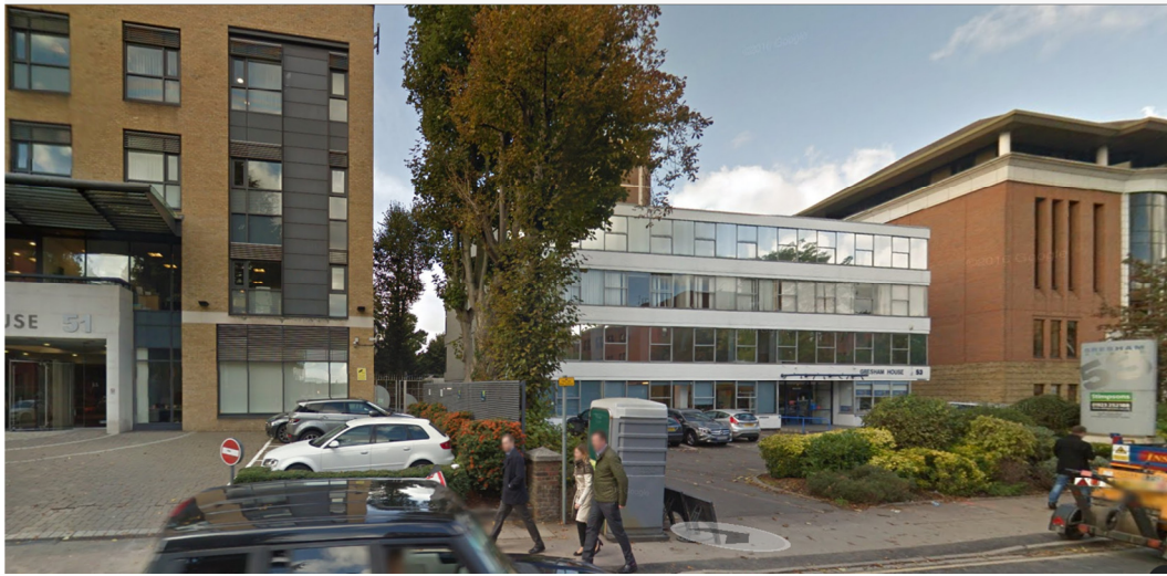
The existing building
